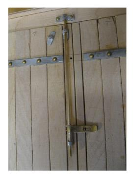
Mark out the required length of the latch bolt allowing for the bolt to pass into the top latch keep, mark out the position of the bottom keep allowing for the bolt to drop down to clear the top latch, solder the brass locking tab to the brass rod. Position the top mounting plate on the door for the bolt to pass through into the top latch plate. Locate and fix the bottom keep in place and fix the brass nut on the end of the bolt to retain this in place
