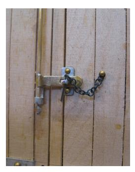
With the bolt in the top keep locate the latch plate to the door and add the chain and split pin to close this off.
