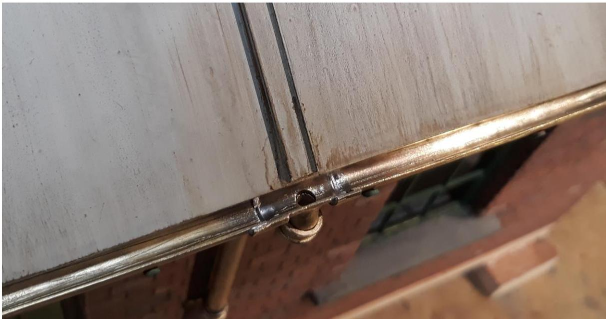
The RW7 Offset bend will allow for adjustment on the position of the downpipe in relation to the gutter outlet – the offset is designed for a fascia set at 18mm off the building measured from the wall to the outside edge of the fascia
