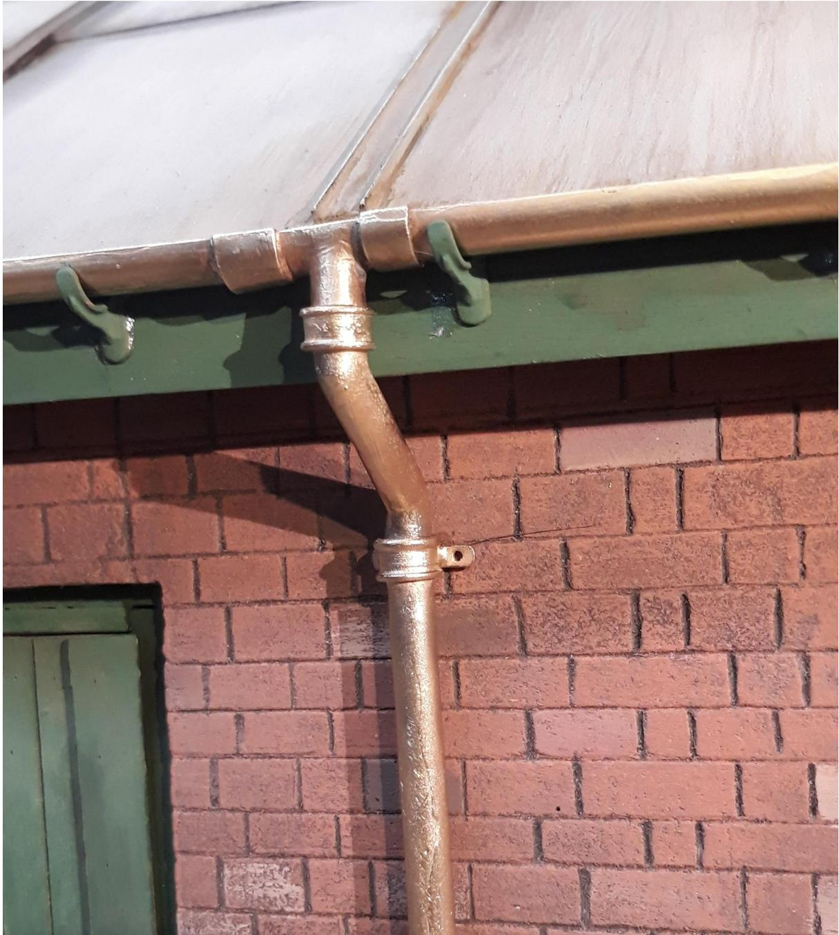
It's a good plan to work out the fascia bracket locations and fix these in place making sure that the gutter tucks in under the roof overshoot – once the brackets are fixed in place its best these are all painted along with the gutter and downpipes, once these are dry then carefully fix in place with epoxy to the brackets and line up the downpipe assembly
